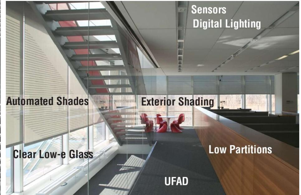
2 years of LBNL testing in a 500 m<sup>2</sup> mockup was used to refine and spec the final design
