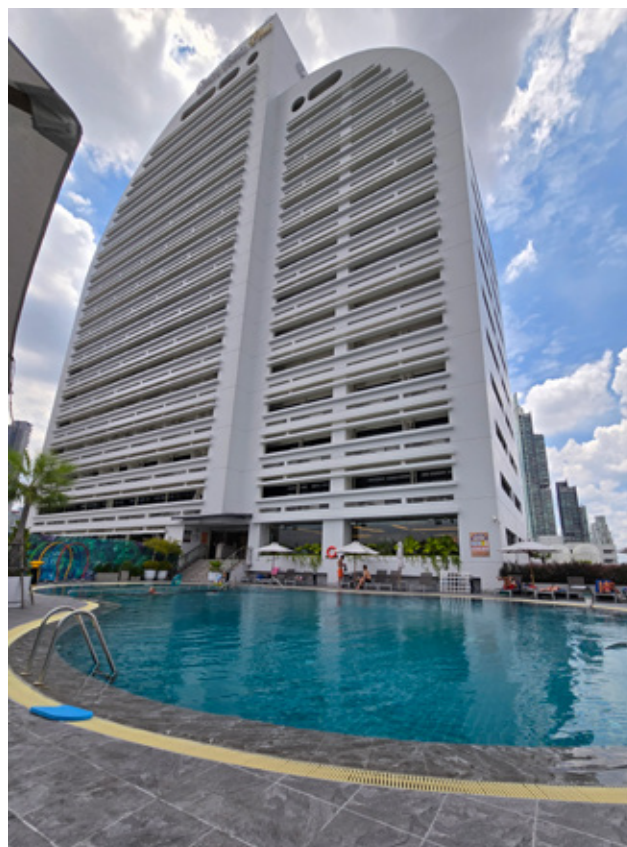
Centre Point Plus Hotel Silom
