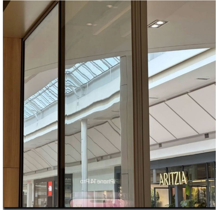
Fig. 3 - Mix of draw lines, edge and lamination distortion.
