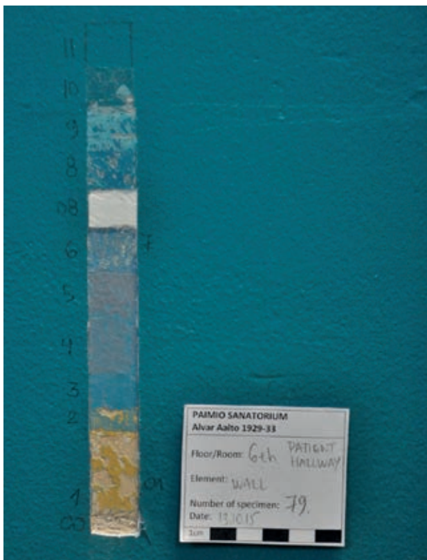
Uncovered paint layers in a corridor. Photo: Nina Robin.
