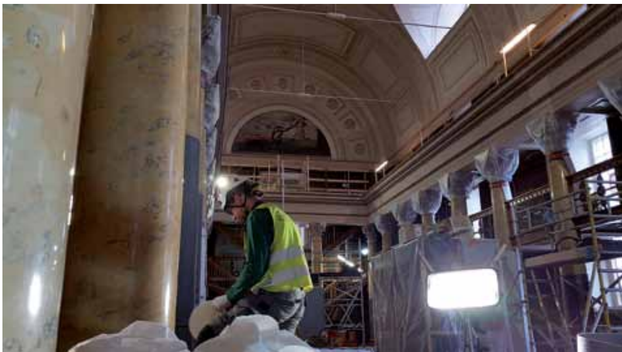
1. Interior of The North Hall. Conservator Teemu Kajaste working with the scagliola repairs.
