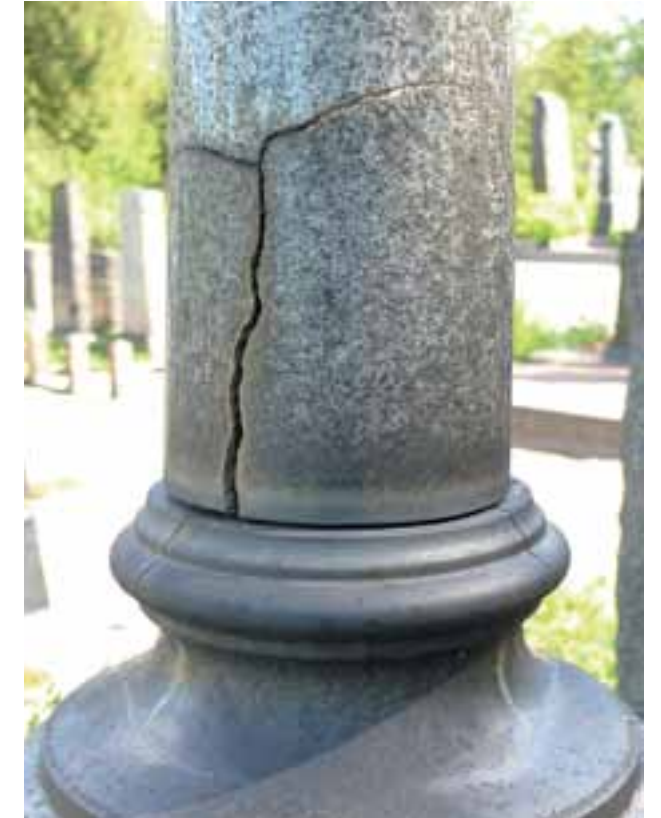
6. Many cracks on a marble grave monument due to freeze-thaw and corrosion of the dowel.
