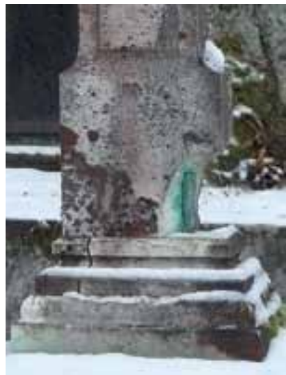
3. Dry stone wall type of grave monument at the final stages before collapsing.
