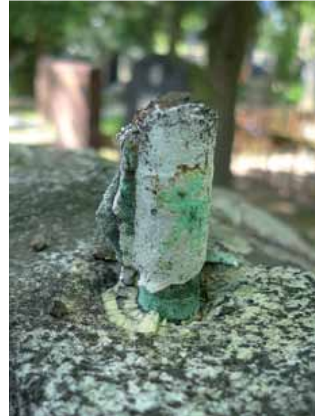
5. Exposed copper dowel.
