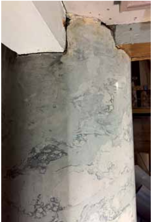
2. Cleaned area at the Cupola Hall column.
