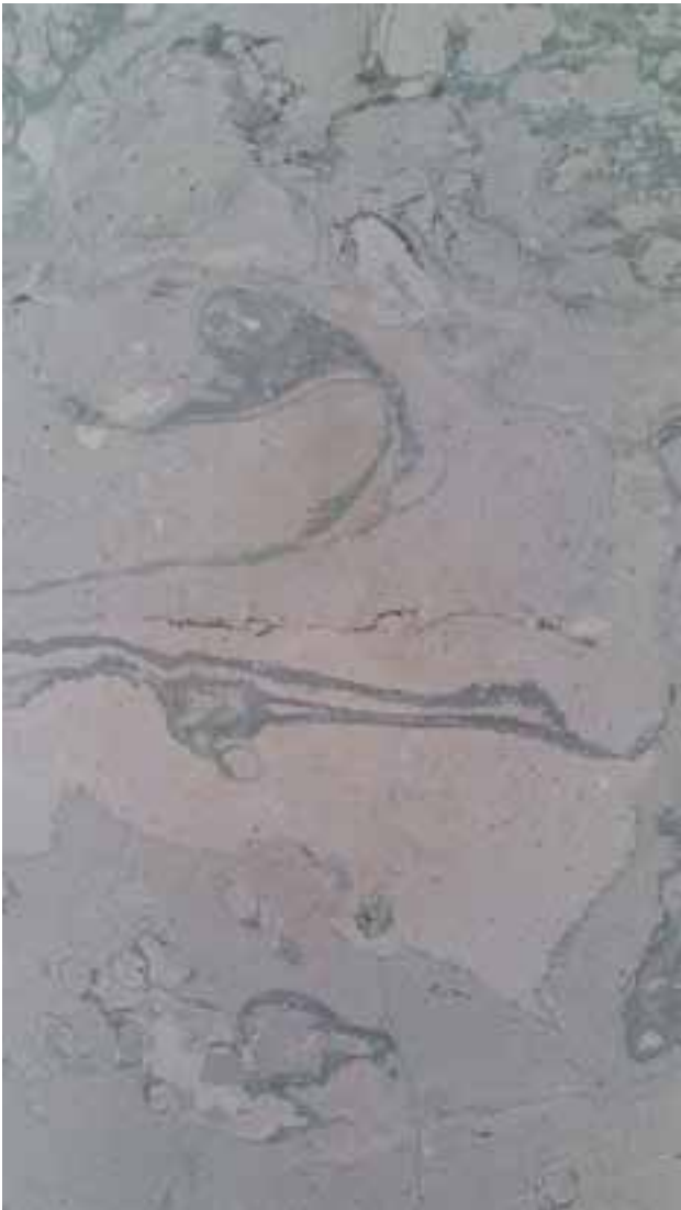
6. Missing area after patching with Modostuc and watercolours.
