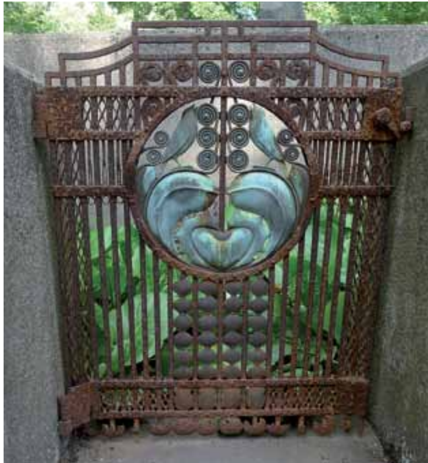
17. Ornate art nouveau gate at advanced stage of rusting, showing handicraft and mixture of materials.
