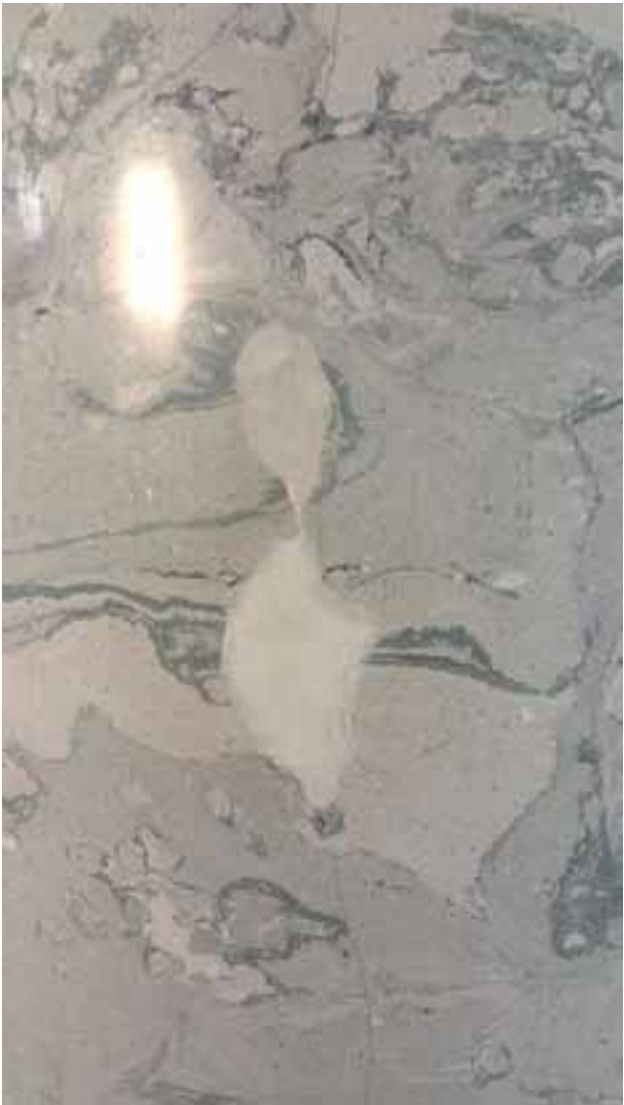
5. Missing area before patching.
