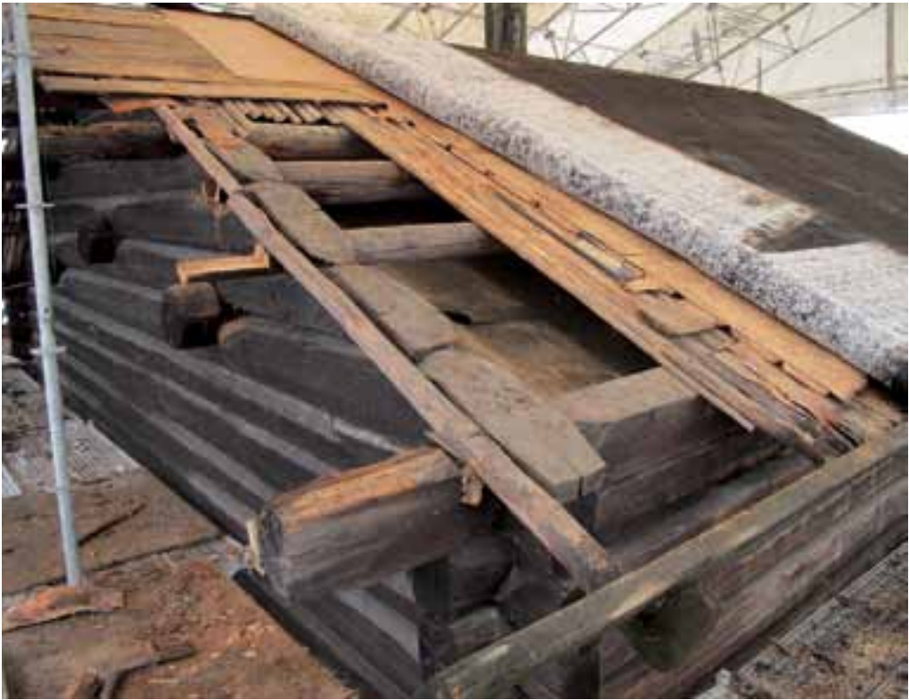
2. Roof layers under restoration.
