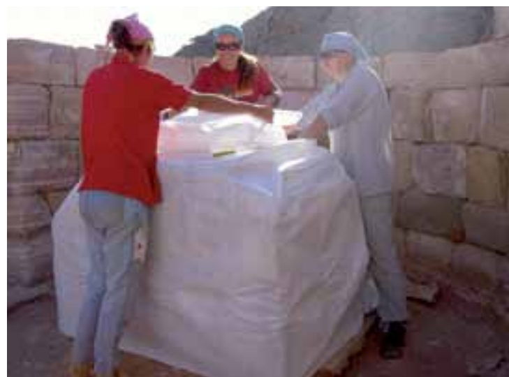
5. Conservators covering the plastered altar with geotextile. Photo: Susanna Eklund 2005.
