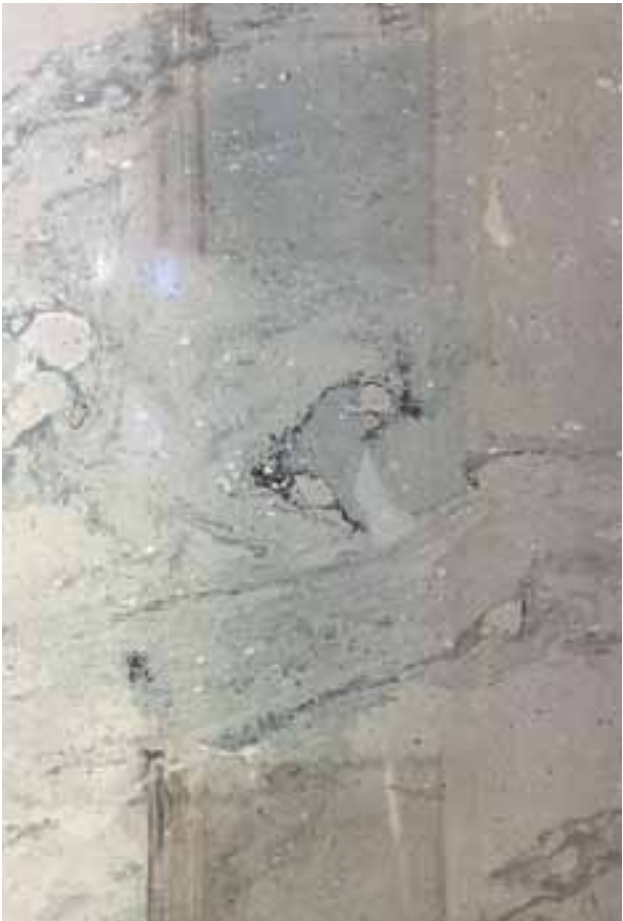
3. After cleaning one of the railings needed to be removed. Area shows the difference between cleaned and untouched scagliola.
