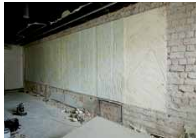
6. Mural covered by layers of prophylactic fabric prior to demounting. Photo by Peeter Säre.
