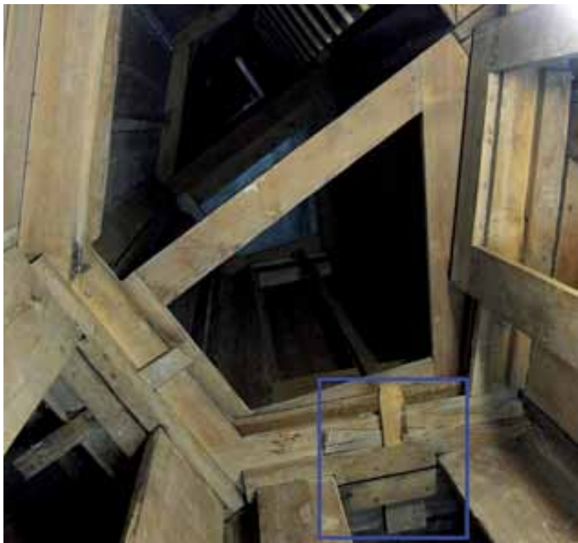
8. A wedge mortise and tenon joint (blue colour) on a frame of a module inside the altarpiece. Photo: Disent AB.
