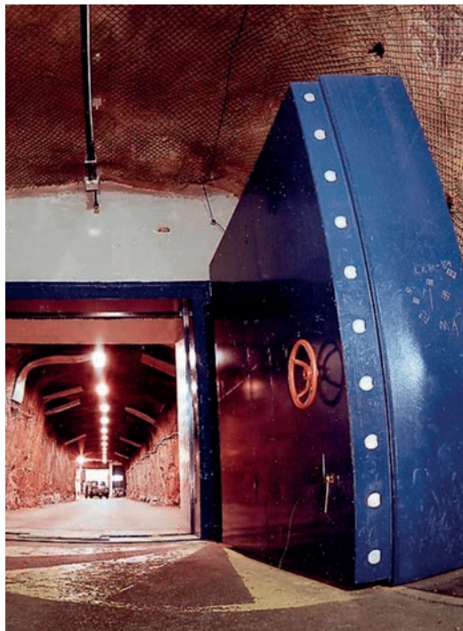
One of the three 10-tonne blast doors in the Underground Complex, Canadian Forces Base North Bay.
