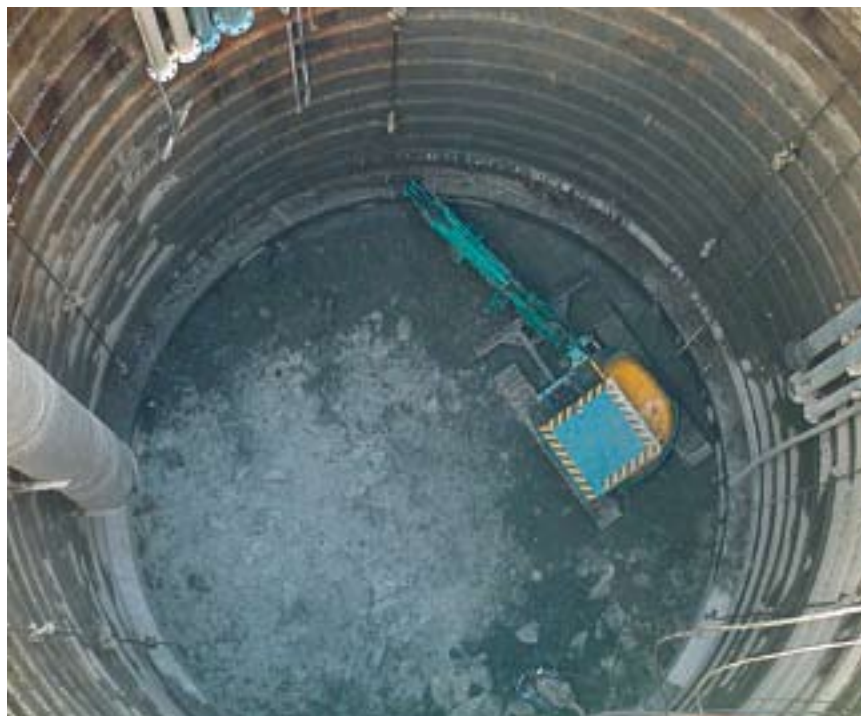
Shaft construction at Mizunami URL (Photo:NUMO archive)
