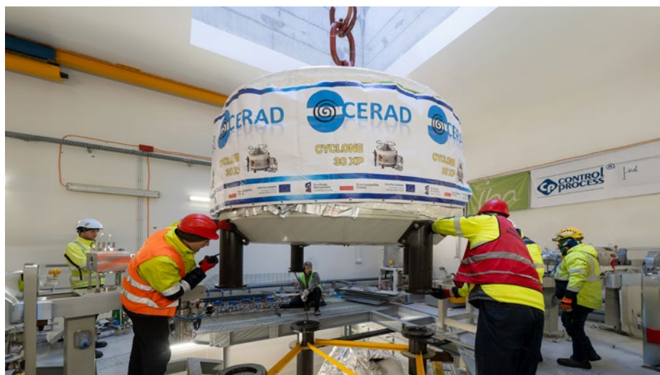
Installation of the IBA Cyclone 30XP cyclotron at the CERAD centre, NCBJ.
