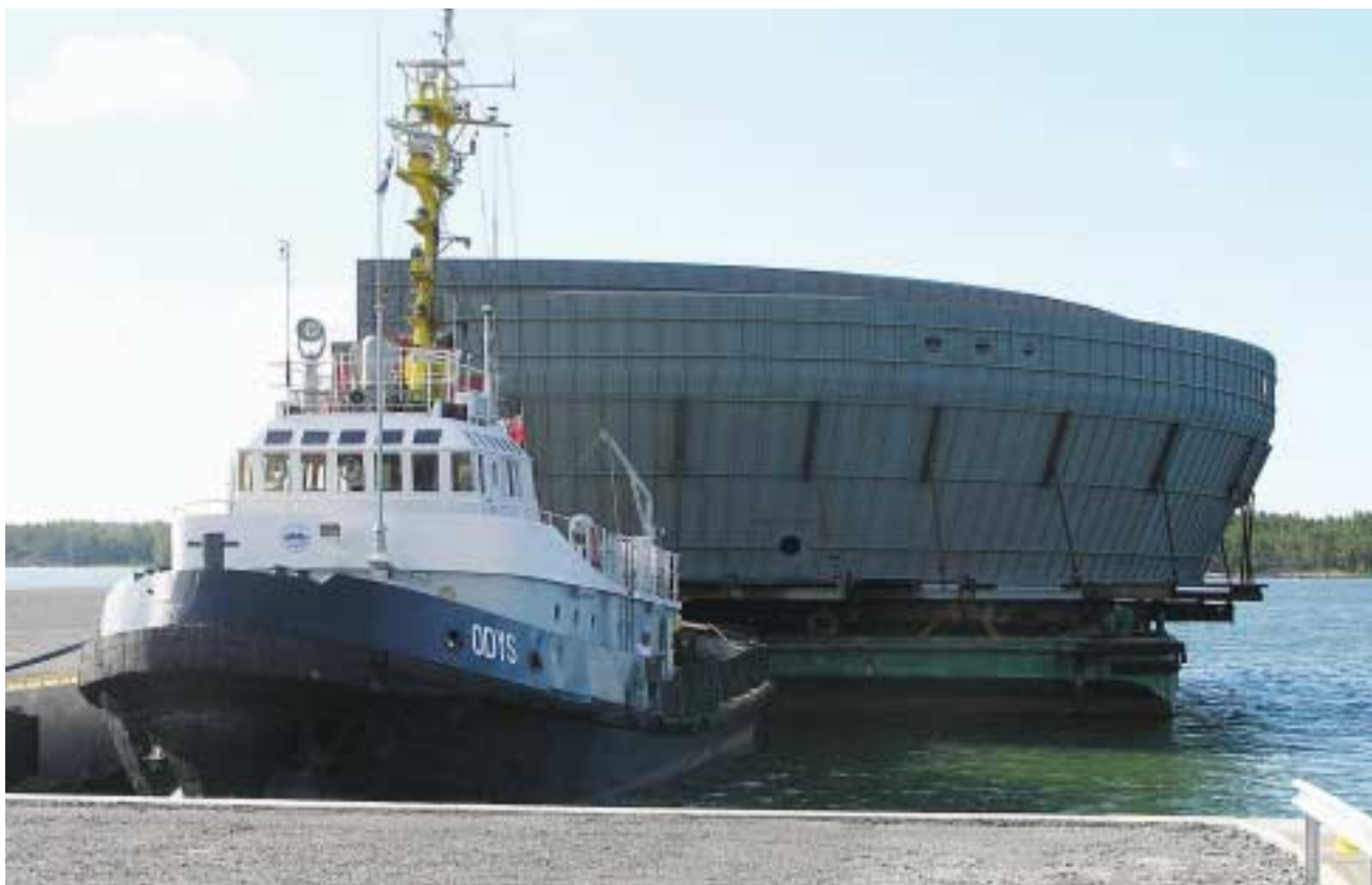
On July 15, the first sections of the metallic liner for the inside of the reactor containment building arrived by sea at the Olkiluoto 3 construction site.
