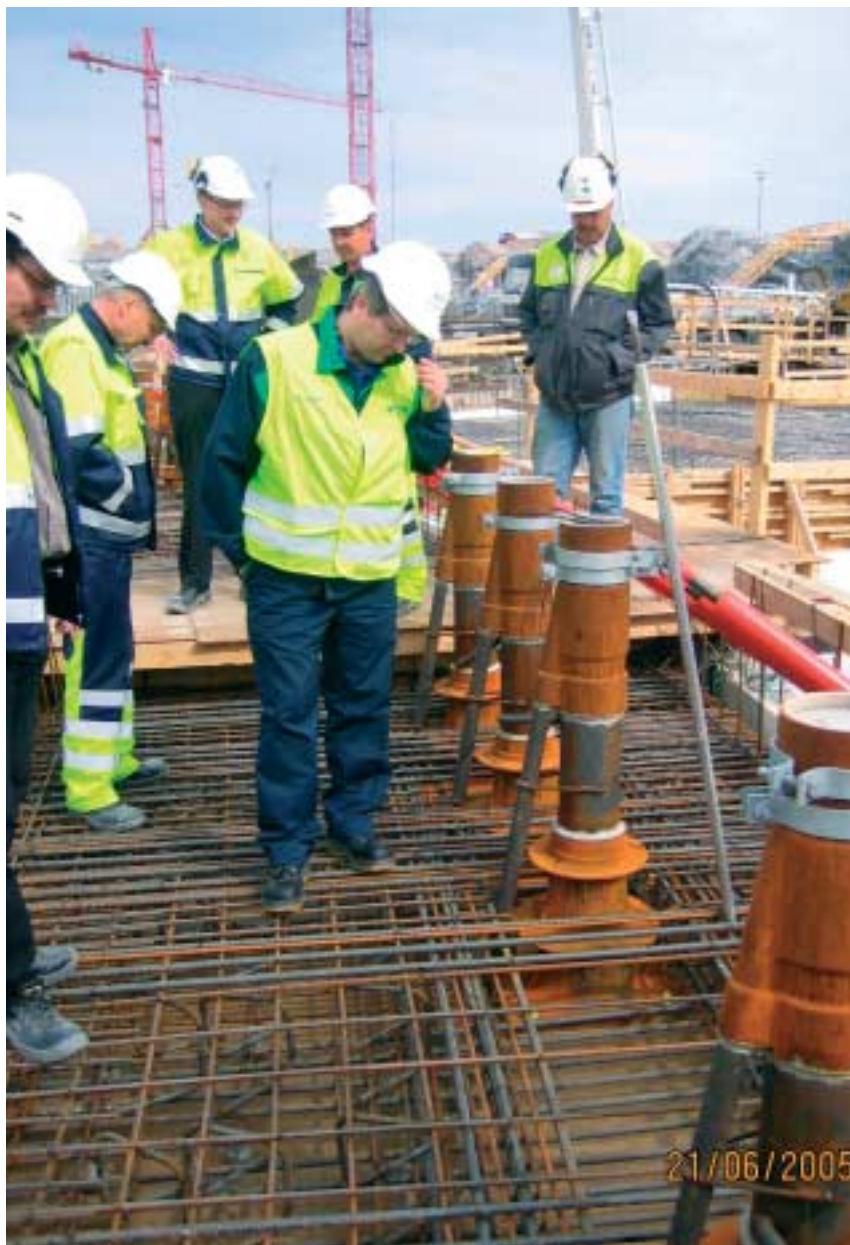
On-site inspection of OL3 reactor basemat structure.
