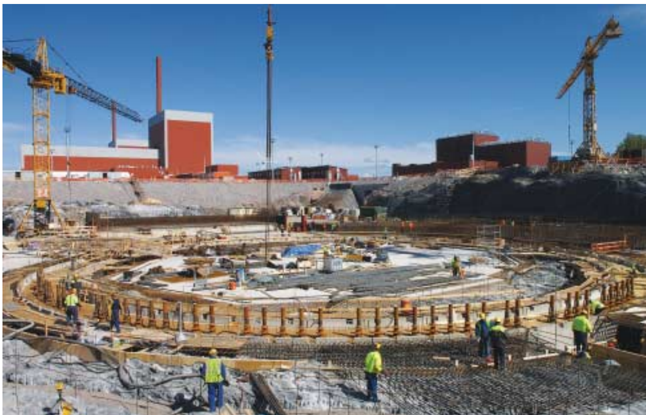
Summer 2005: Situation on site looking at the basemat of the reactor building.
