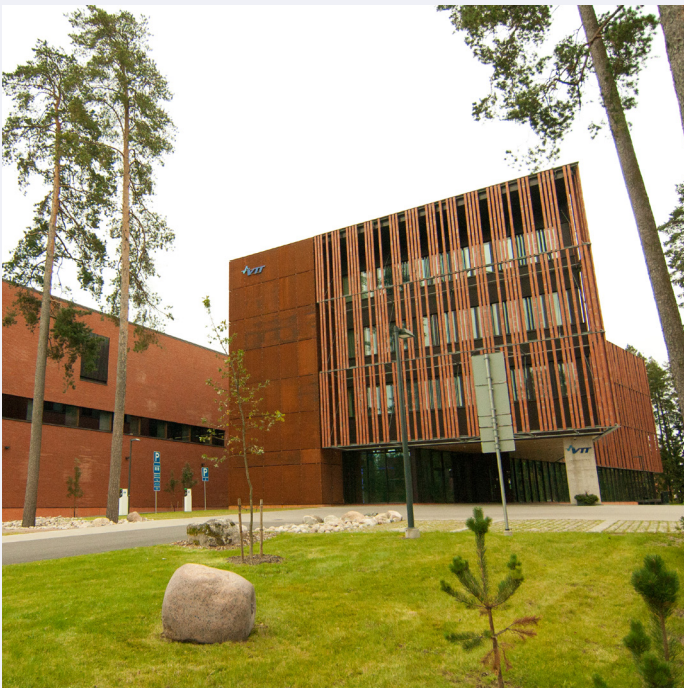
Figure 4. Two years after the site work was initiated, the office wing of the new facility was ready for move-in, and in early May 2016 the laboratories were also turned over to VTT.
