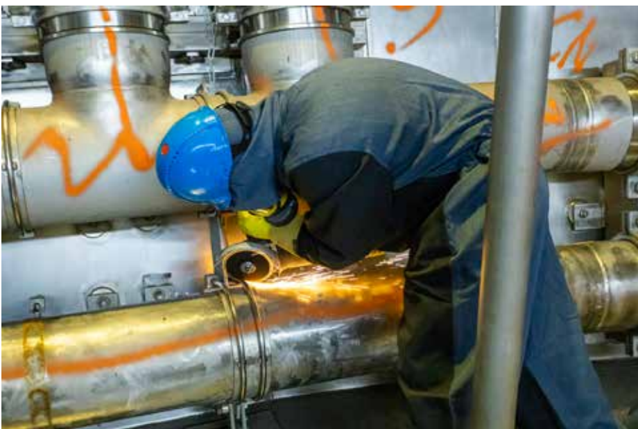
Oskarshamn unit 2 wet-well equipment being dismantled (photo: Uniper).
