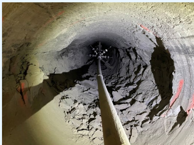
Figure 4. Example of waste disposal tunnel studied in OPTI work package for optimisation and closure.
