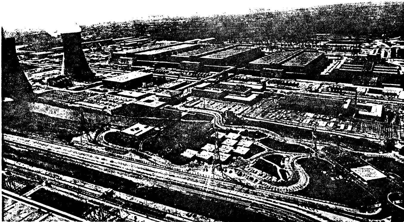
SLIDE 12 : EURODIF PLANT
