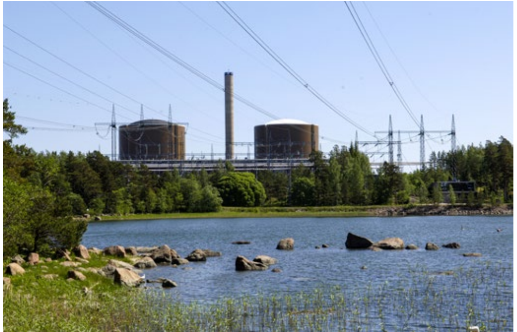
The Loviisa nuclear power plant (Fortum).
