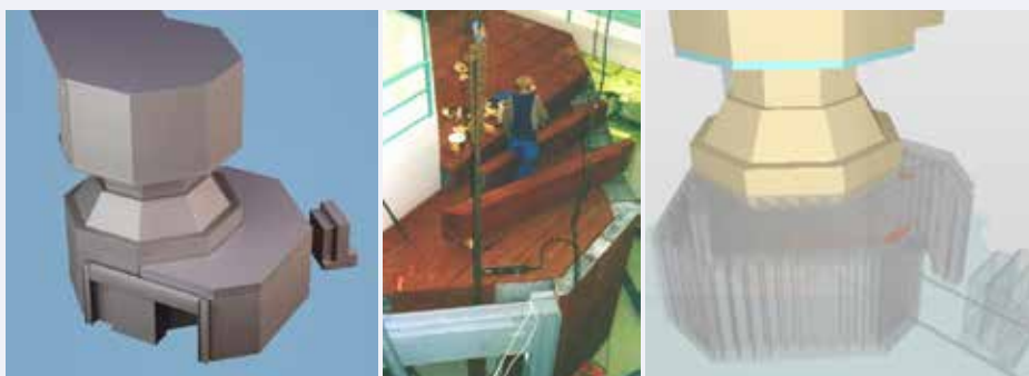
Figure 1. A shielded irradiation room was built around the BNCT neutron beam using heavy concrete filled steel bars (photo from construction phase: VTT, 3D virtual model: Sweco).
