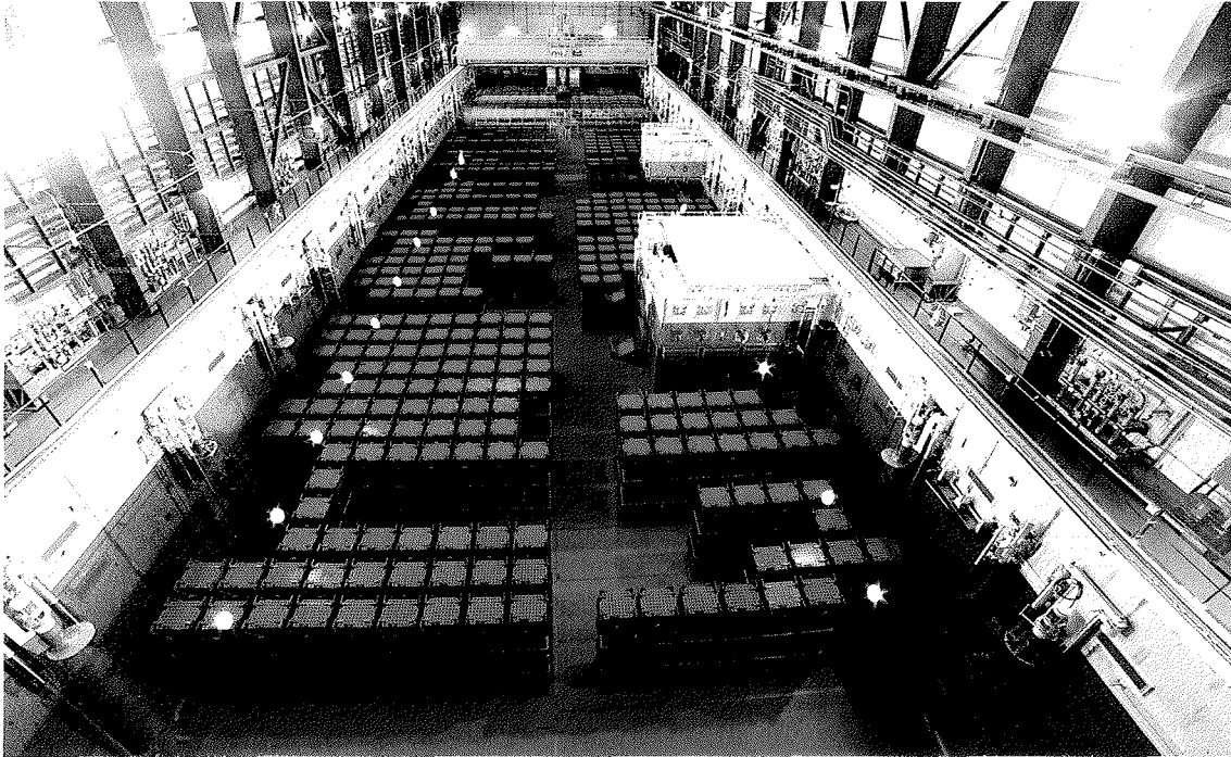
Spent fuel pool at La Hague reprocessing plant (Photo: Cogema).
